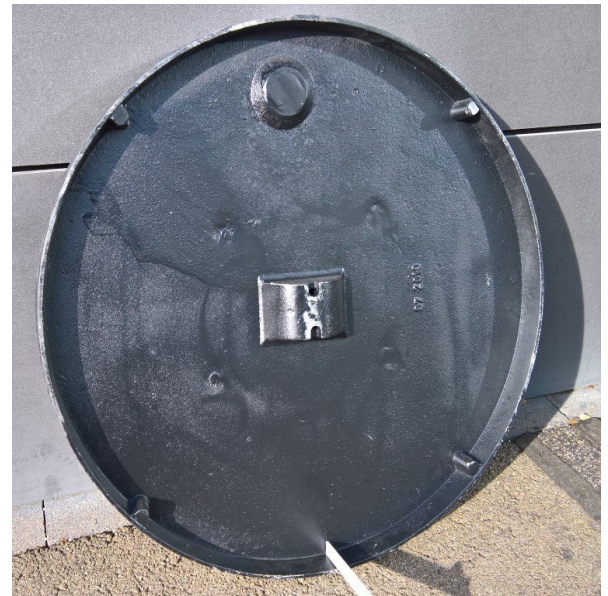
Fig. 2 Bottom view with edge upstand
